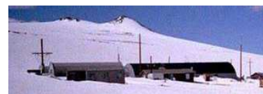
FIG. 9: Barcroft Station at 12,500 ft
